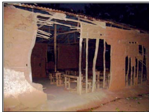
Figure 3: Renovated and non-renovated classrooms at Bogamachuko Primary School
