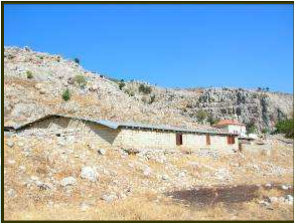
These old sheds will be demolished and replaced by the Eco-Lodge
